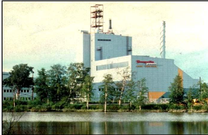
80 ton per day Gasification Pilot Plant in Tampere, Finland using biomass & coal
